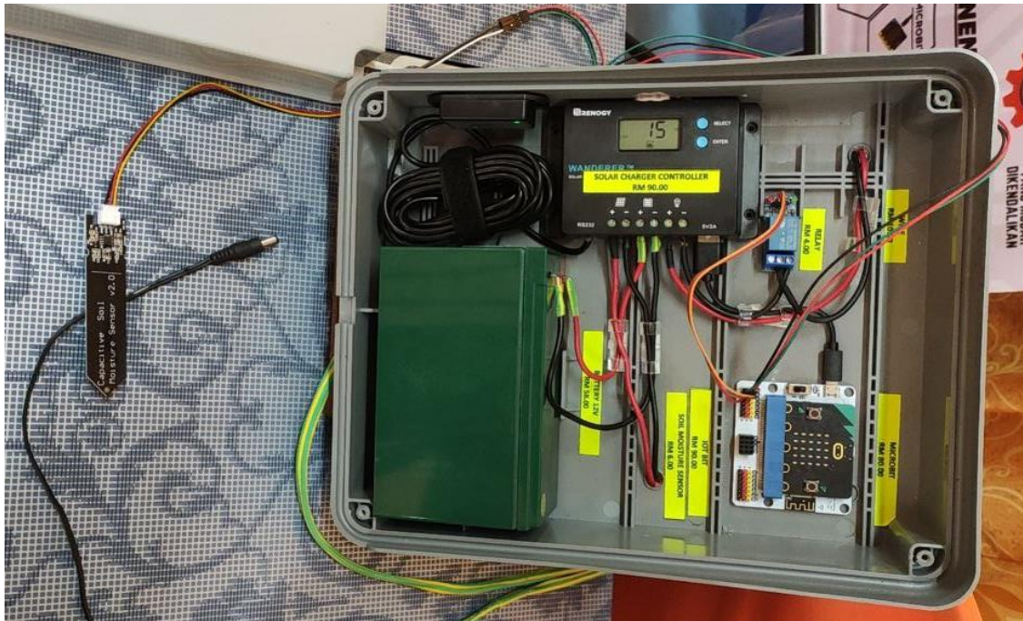
(The process of upgrading the system)
