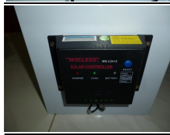
The battery is place in a box and the solar controller is attached outside the box.
