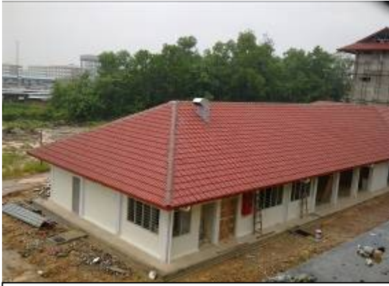
School experiencing Flooding
